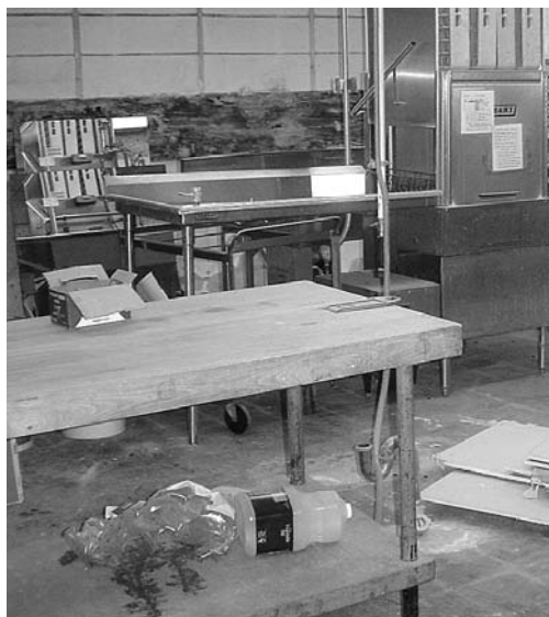
Members hope to have the church kitchen, shown above in the wake of the flooding, rebuilt by Easter.
