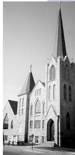
Narthex addition on far left, after its completion by Mission Builders earlier last year,
